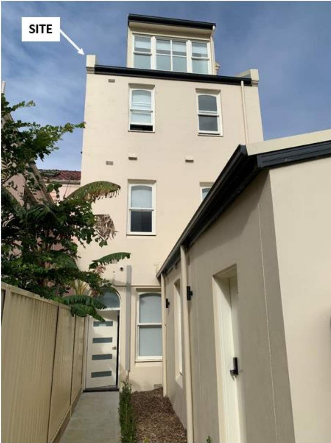
Figure 5: Northwest elevation and rear wing of existing terrace viewed from the rear yard
